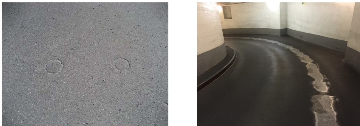
Figure 1.2 Example of damage in the form of sink marks for mastic asphalt (left hand side) and wear for plastic-based systems (right hand side)
