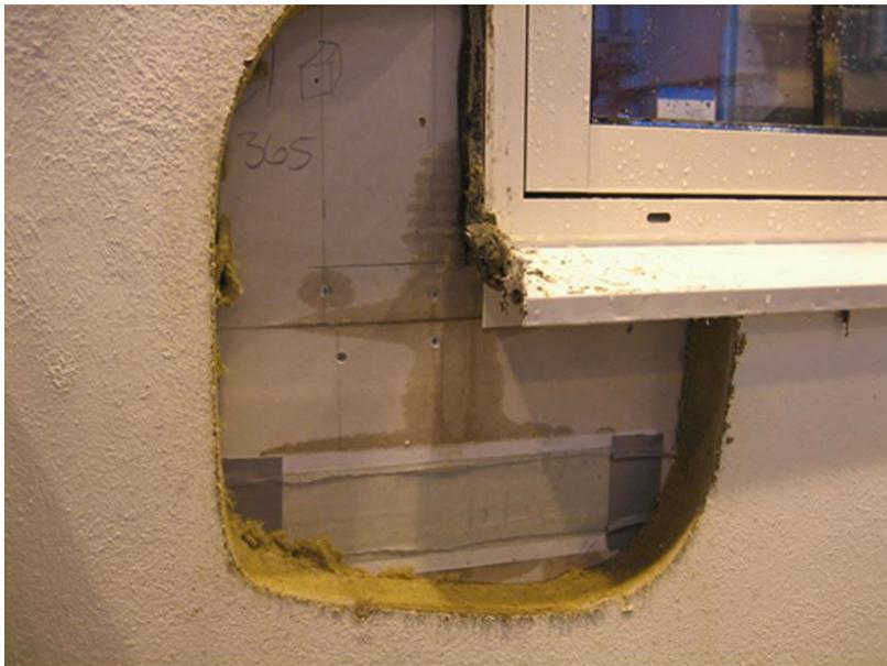
Figure 11. Rain leakage at the corner of the window-wall interface in an ETICS façade (photo from after the measurements were finished and the wall was opened). The material behind the plaster and insulation board is in this case moisture retaining, which should be avoided.
