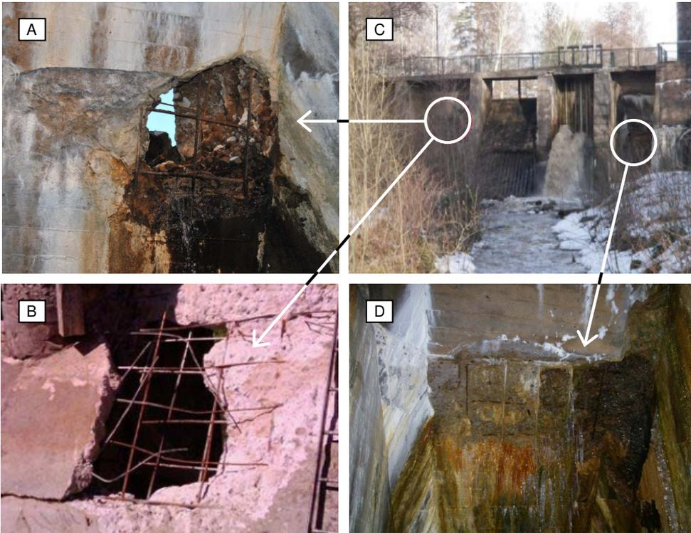
**Figure 3-3. A severely damaged buttress dam (C). The concrete cover was missing in some places in the vicinity of water leakage through cracks on the downstream face (D). A hole appeared in the flat slab in another place and water escaped flushing away loose pieces of concrete (A-B). Only the reinforcing steel was left.**
