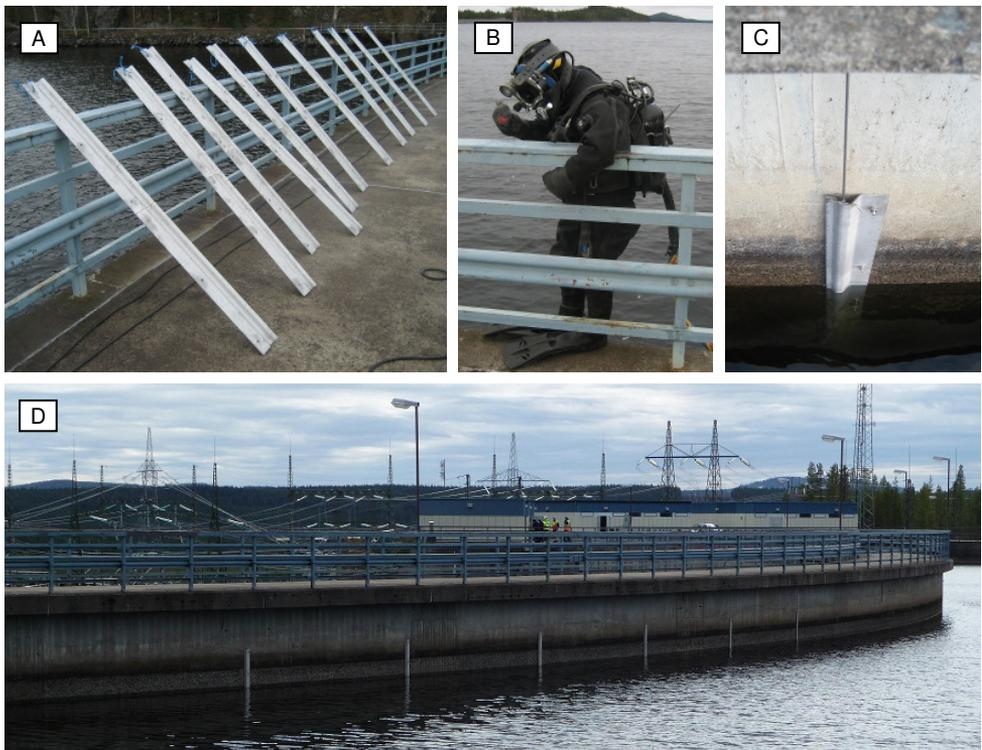
**Figure 7-1. Stainless steel profiles (A) to be mounted by divers (B) on the upstream face of the arch dam (D) at Vargfors power plant. The top 0.5 m of the steel profiles are above the maximum water line (C).**
