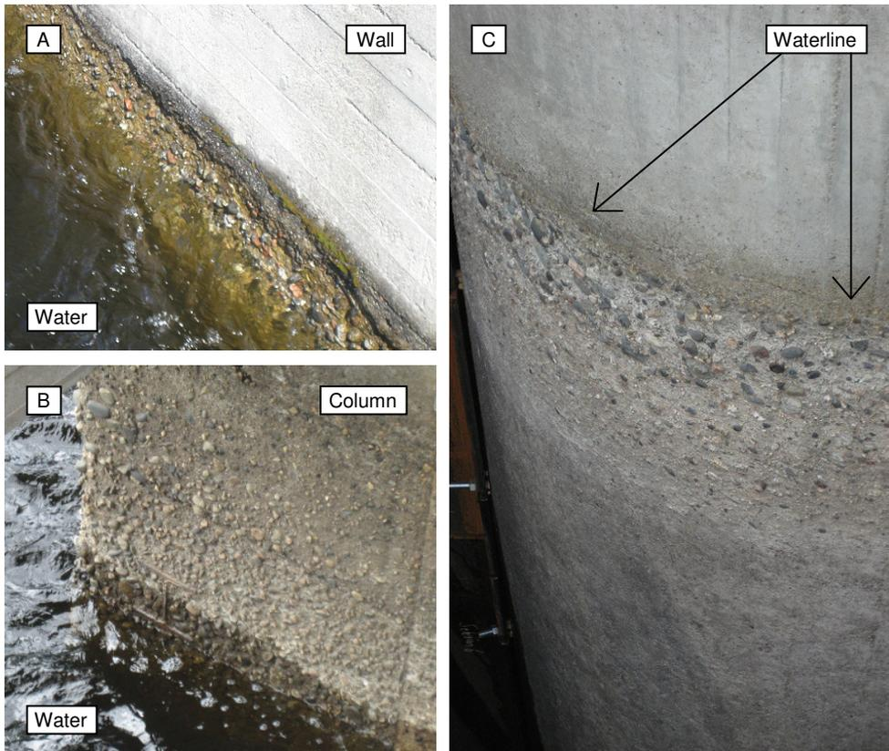
**Figure 3-1. Photos of damage to the concrete surface at the waterline of hydro power structures. The photos A and C are taken on the upstream side, whereas the photo B is taken on the downstream side of the dams.**
