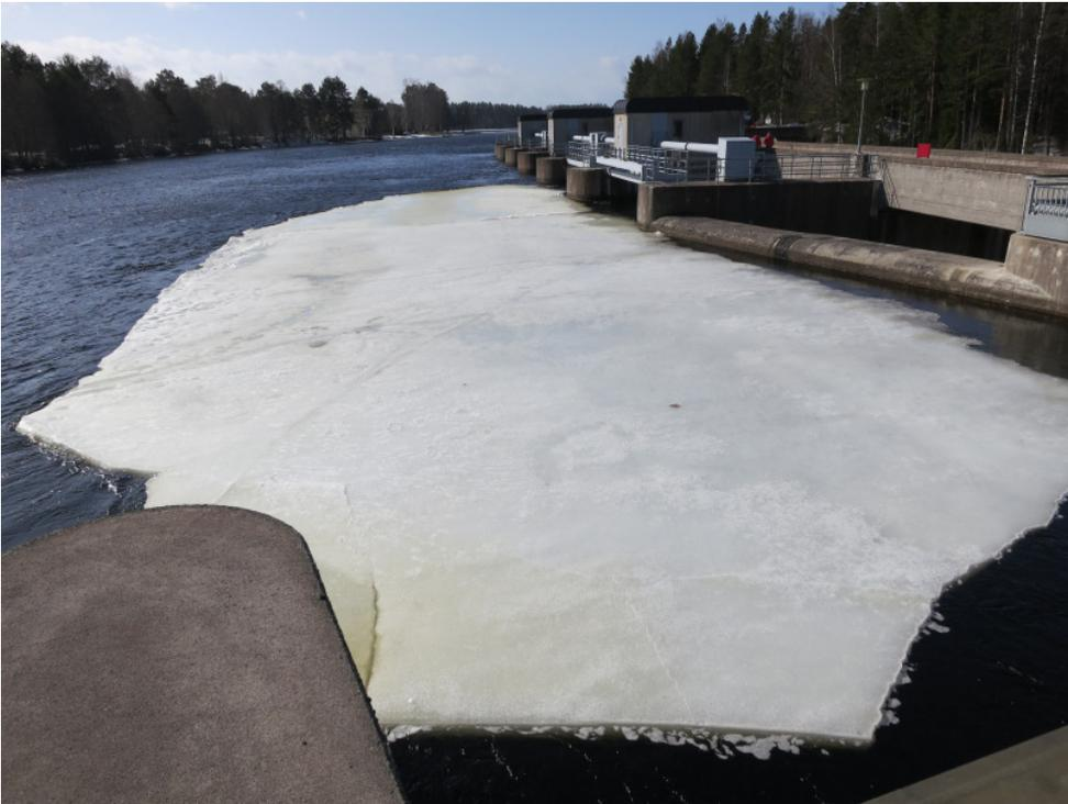
**Figure 2-9. Ice floe pushing against a bridge column in spring.**
