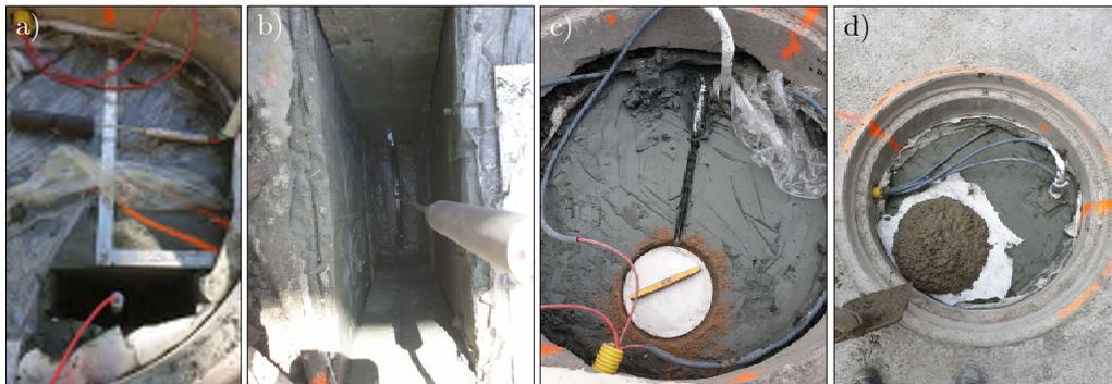
Figure 4.27: *Installation of total earth pressure cells within one of the three well rings; a) and b) cell installed to measure horizontal earth pressure perpendicular to SPWs, c) cell to measure vertical earth pressure and d) careful pouring of concrete over instruments as final part of the installation.*
