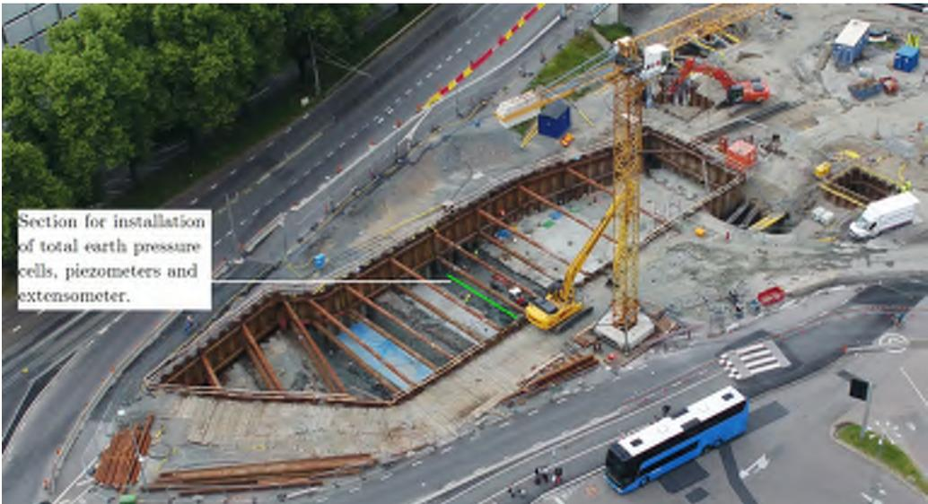
Figure 4.7: *Excavation to final depth in studied section. Photo from drone on June 26<sup>th</sup> 2019.*
