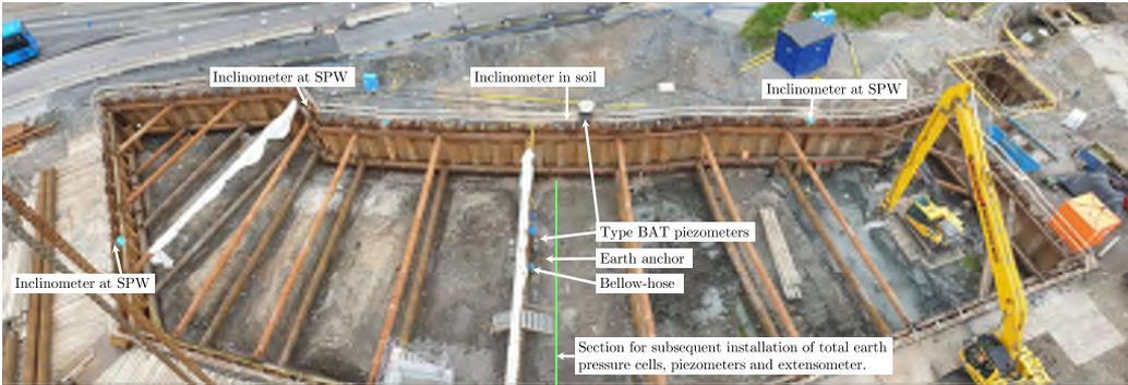
Figure 4.6: *Excavation to final depth started from north (right in the photo) on May 29<sup>th</sup>. Studied section including instrumentation is highlighted. Photo from crane on June 5<sup>th</sup> 2019.*
