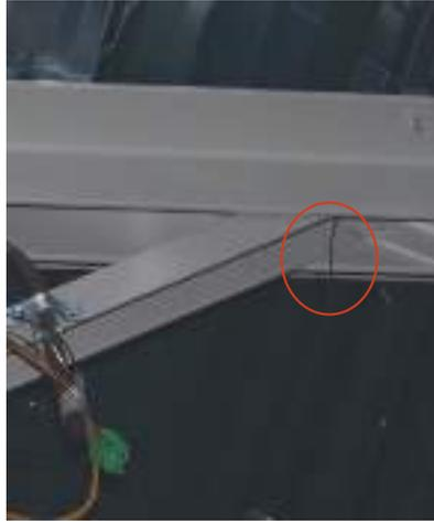
*Figure 7. Thermocouple mounted 100 mm below the upper chord of truss F2.*
