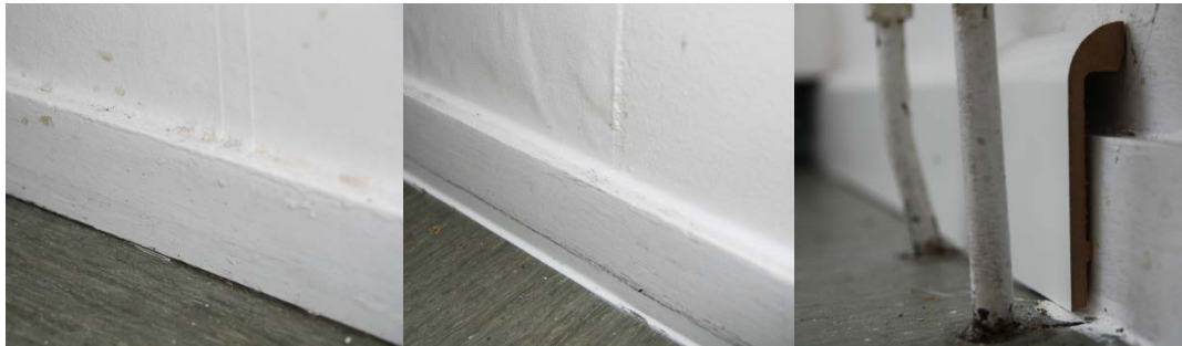
Figure 3.1 Left: original state of skirting board. Middle: skirting board when sealed. Right: part of “Renoveringssockeln” mounted.
