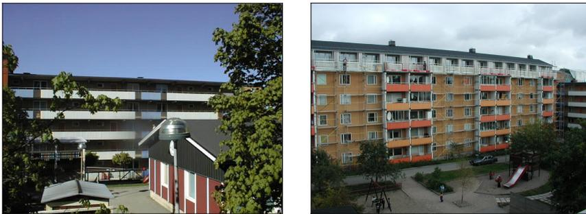
**Figure 5: Modular over roofing, the Husby project. Before and after one floor extension is placed on the roof of the existing building**
