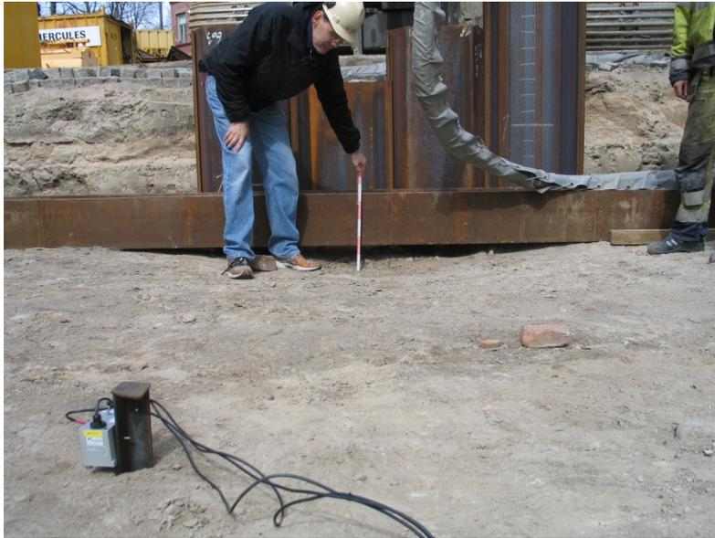
**Figure 13.** Observed settlements due to the sheet pile driving.
