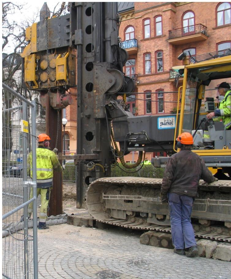
**Figure 3.** Driving equipment used in trial sheet piling
