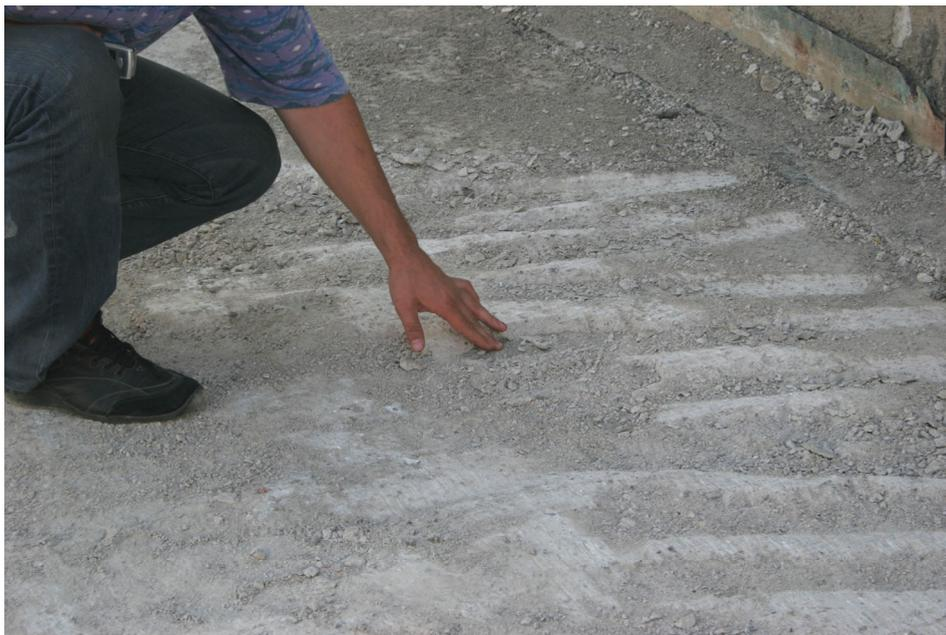
*Figure 5.19 Typical surface condition of area 2 and 3 after removal of the overlay concrete.*
