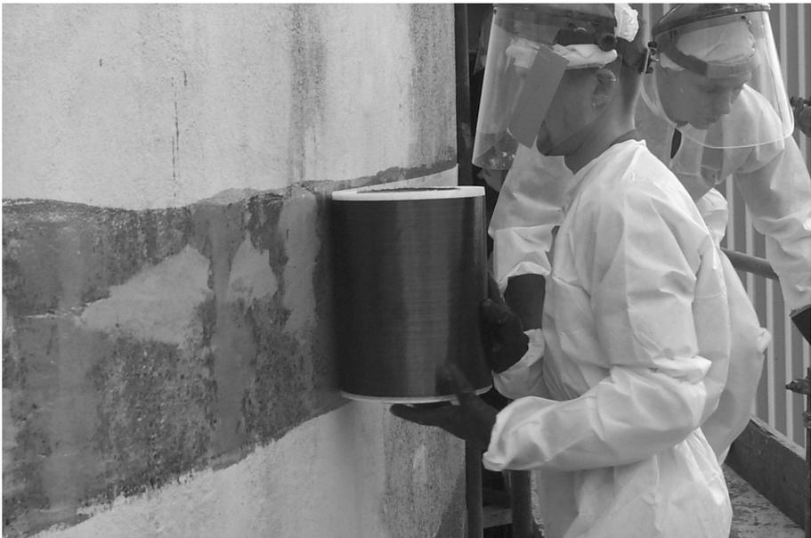
*Figure 2.6 Strengthening of a concrete silo with composite wrap system.*
