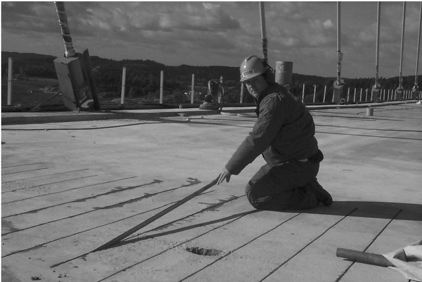
*Figure 2.8 Strengthening of a bridge joint with BPE<sup>®</sup> NSMR system.*
