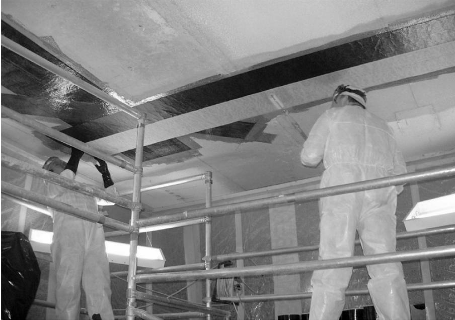
*Figure 1.1 Strengthening with CFRP sheets before making an opening for a ventilation duct in an existing slab due to changed functional requirements. Photo Björn Täljsten (2000).*
