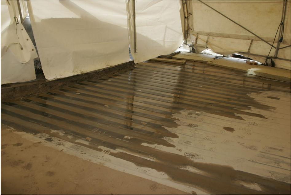
*Figure 5.17 Flooded strengthening area.*
