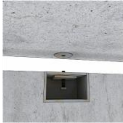
Figure 12 Intermediate floor element supported on wall element, Consolis (2007).
