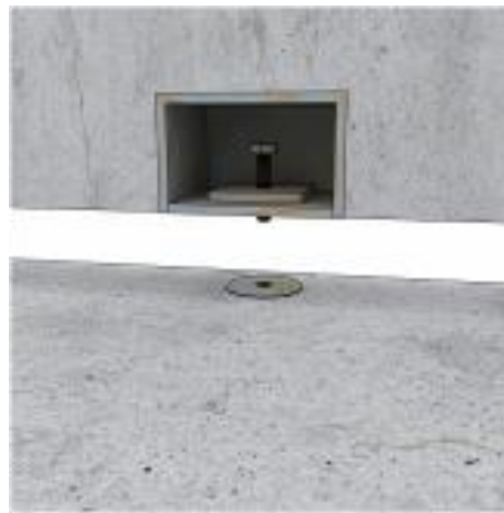
Figure 13 Wall element supported on floor element, Consolis (2007).
