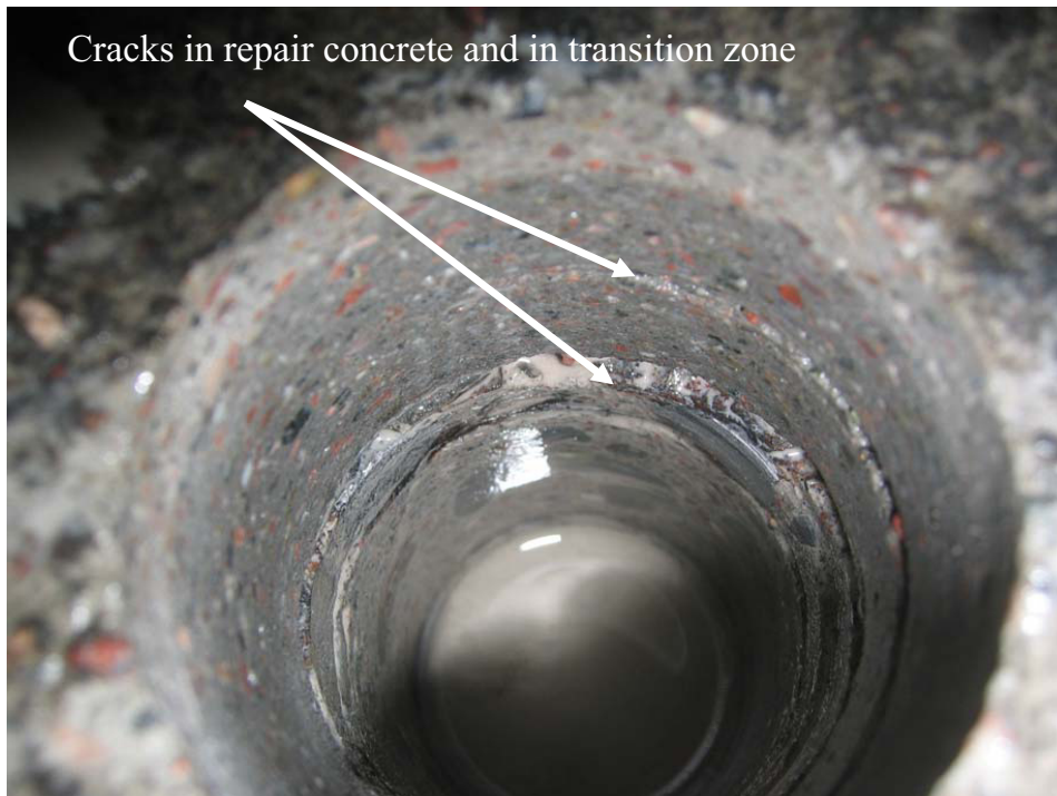
Figure 8. Sample hole in a concrete repair. Note the horizontal cracks.
