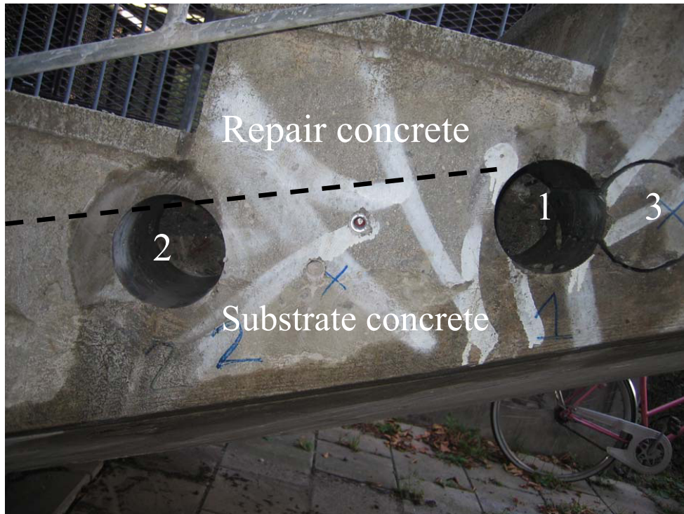
Figure 5. Repair concrete on the top and substrate concrete beneath. Concrete cores 1 and 2 were drilled out.
