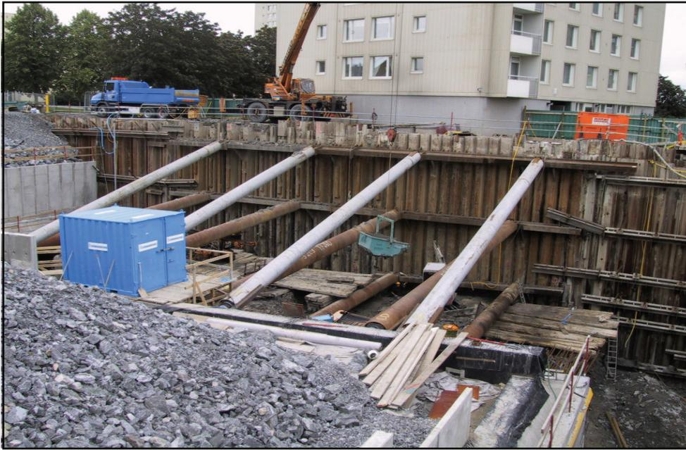
Figure 4.2 The sheet pile wall with supporting system of struts and anchors at the residential block Asplången (Carlsson et al. 2004).
