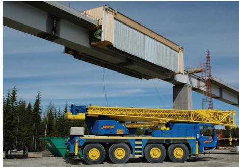
*Figure 6.5 Weather protection for casting of concrete after launching, Nätraån, Sweden.*
