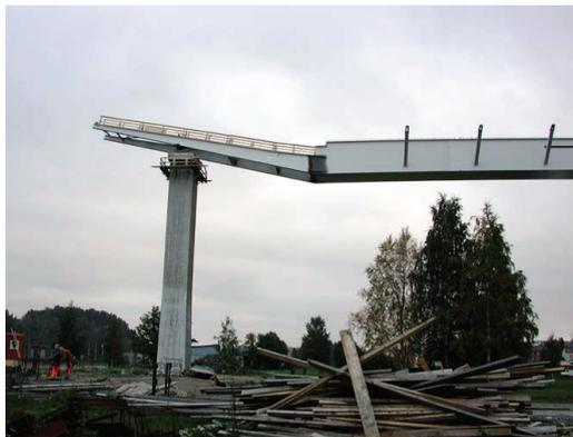
*Figure 6.2 Bridge launching with a launching nose in the front, outside Sollefteå in Sweden.*
