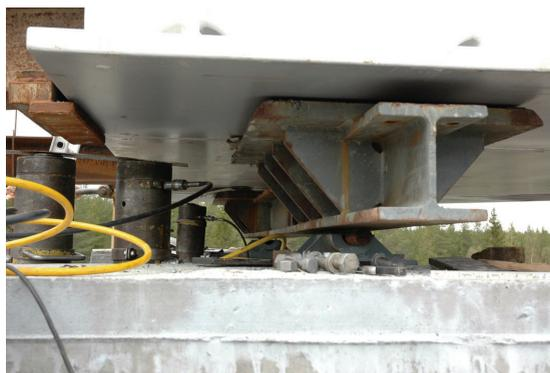
Figure 6.4 Launching shoe of the slide bearing type at Nätraån, Sweden.
