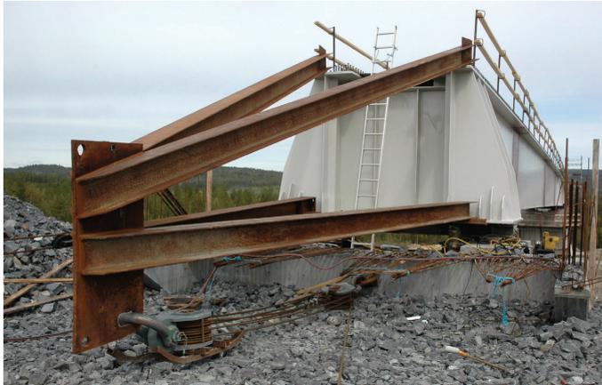
Figure 6.3 Wire system used to both hold and push the bridge girder over Nätraån in the north part of Sweden.
