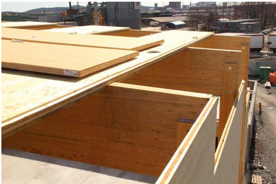
(b) A close-up picture of the CLT-decking.
