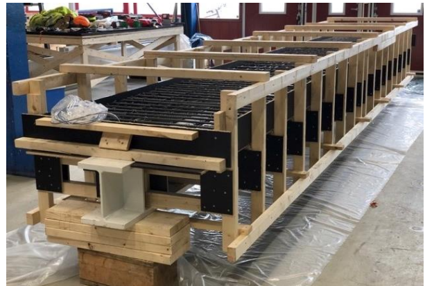
Figure 4. Photo of one of the specimens, before the concrete was cast
