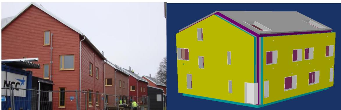
Figure 3. Left: photo of four identical semi-detached houses in Stockholm; Right: simulation model frame of the houses in the IDA ICE software
