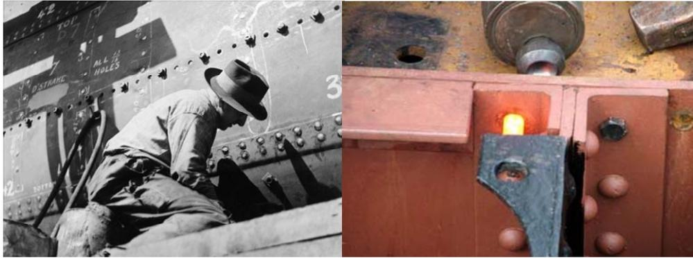
Figure 2.6 On-site riveting
