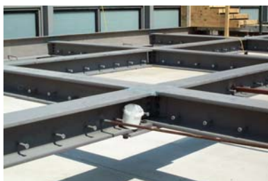
© Sara Jiménez Crown Hall Restoration (2004) - Chicago, USA
