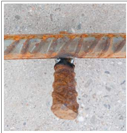
(c) Picture showing welded connection between rebars.
