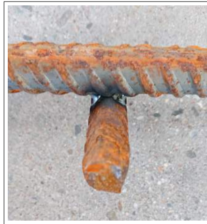
(d) Picture showing welded connection between rebars.
