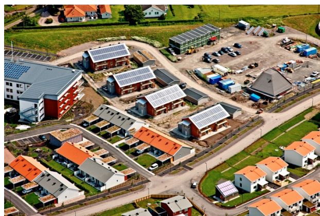
Figure 1: Passive house residential area Vallda Heberg during construction [4].
