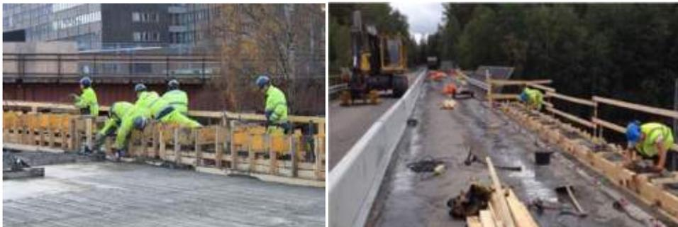
Figure 1: a) Construction and b) replacement of a Type I edge beam
