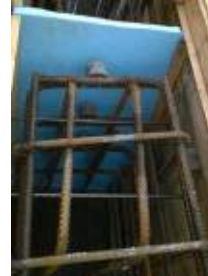
Figure 21: Edge beam in the landscape bridge: a) Cross sectional design, b) Edge beam during construction, c) Formwork layout and d) Joint material (Kelindeman, 2014)
