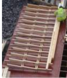
Figure 21: Edge beam in the landscape bridge: a) Cross sectional design, b) Edge beam during construction, c) Formwork layout and d) Joint material (Kelindeman, 2014)
