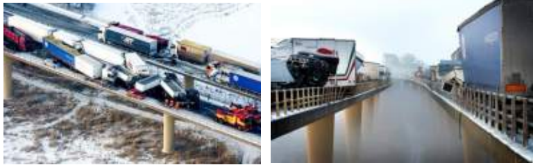
Figure 2: Accident in the Tranarp Bridges (Leprince & Tomas, 2013; Gustavsson, 2013)
