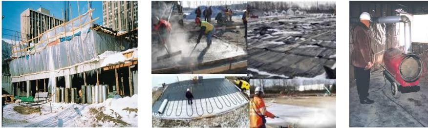
Figure 2: Examples of primitive protection methods of concrete during cold weather, [48]
