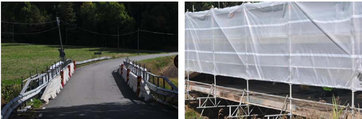
Fig.5.1 Traffic safety measures on the bridge and scaffolding with protection.
