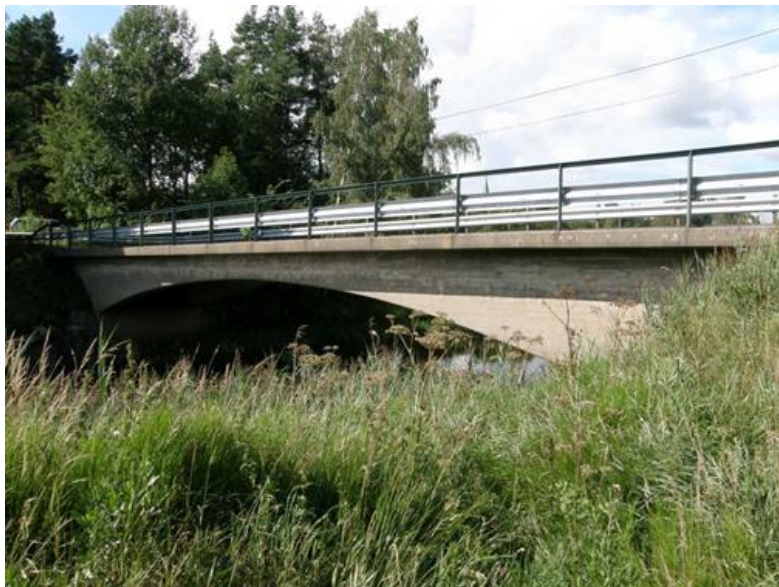
Fig. 3.2 View of the bridge.
