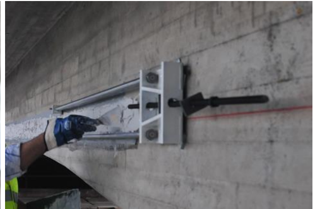
Fig. 5.5 Application of adhesive on the concrete surface.
