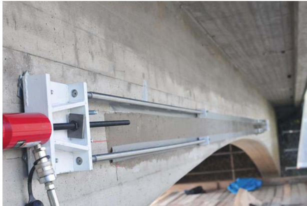
Fig. 5.4 Installation of temporary anchors, guiding bars and pre-stressing jack (red).
